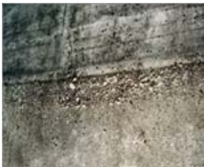
Concrete surface degraded by wastewater
