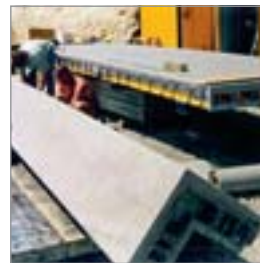
Drinking water reservoir, Schlüsselfeld (D), 1992
