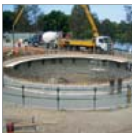
Pumping Station, Gold Coast (AUS), 2007
