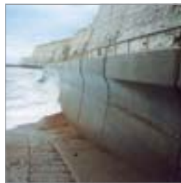
Seawall Brighton (UK), 1992
