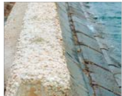
Concrete surface degraded by sea water
