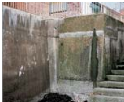
Concrete surface degraded by abrasion and microbiological growth
