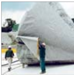
Wastewater Treatment Plant, Munich (D), 1990
